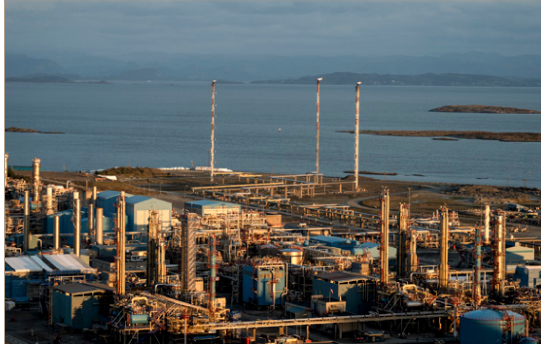
Image: Dry gas is exported to Europe from Kårstø processing plant in northern Rogaland, Norway. Russian knowledge of Norwegian oil and gas infrastructure could become important in a conflict situation.
